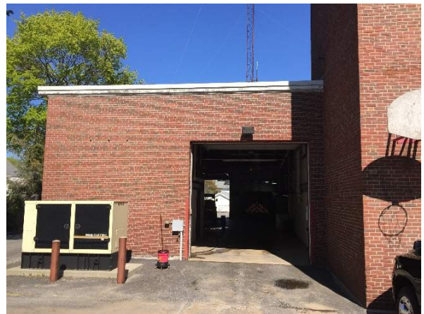
Rear side of Maintenance Bay and generator
