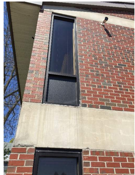
Exterior: replacement windows & precast banding
