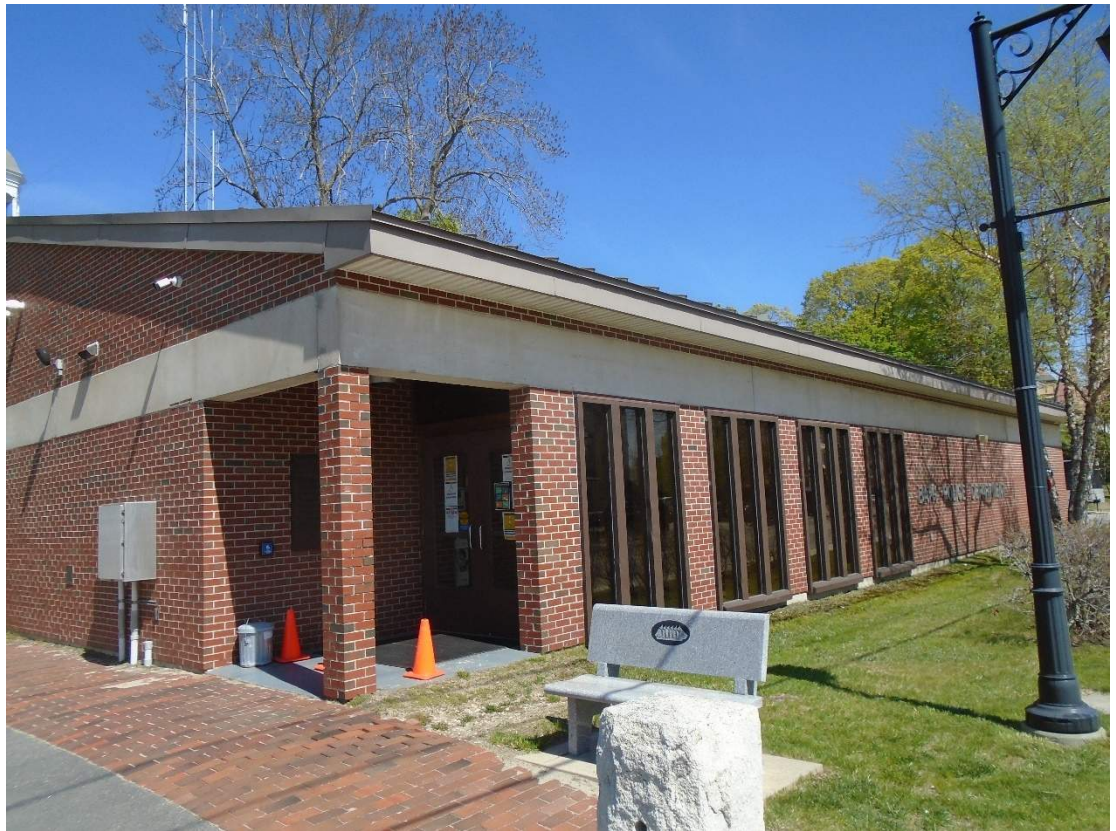
Front Entrance to the Police Station
