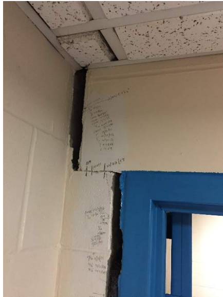
Monitoring measurements of cracking
