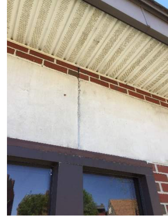
Roof eave and metal coping
