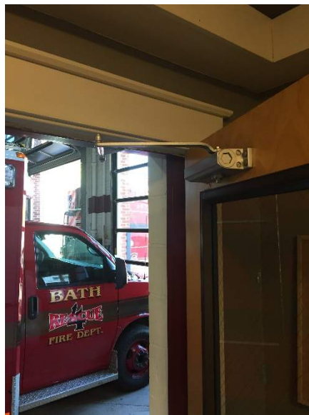
Office space with direct connection to apparatus bay
