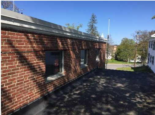
Roof edge and metal coping
