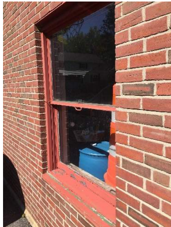
Original copper windows
