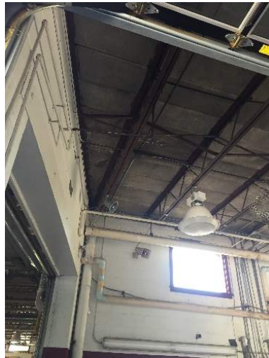
Steel roof framing
