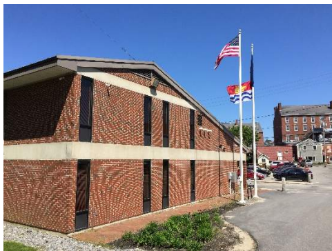
Building Exterior facing Municipal parking
