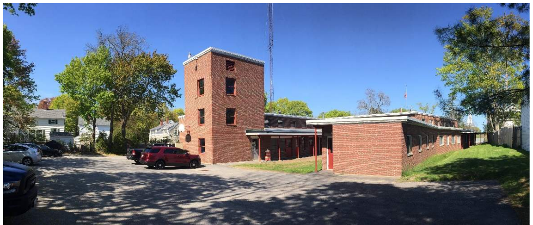
Rear side of building and staff parking
