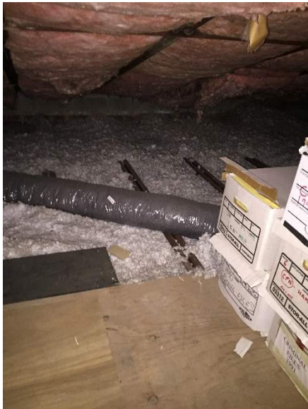
Attic area: storage and HVAC
