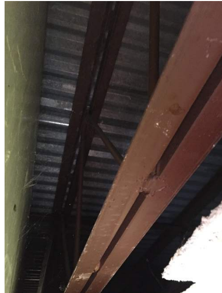
Supported slab framing
