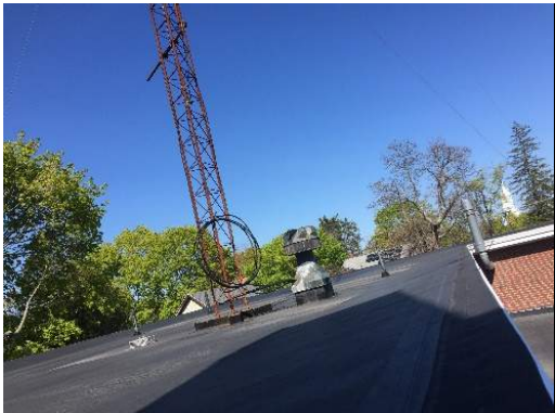
Upper roof over Maintenance and Apparatus Bays
