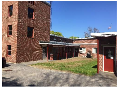
Rear Courtyard and Hose Tower
