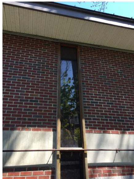
Rear exterior: original wood framed windows
