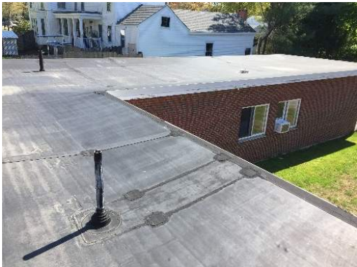
Roof over Day and Residential spaces
