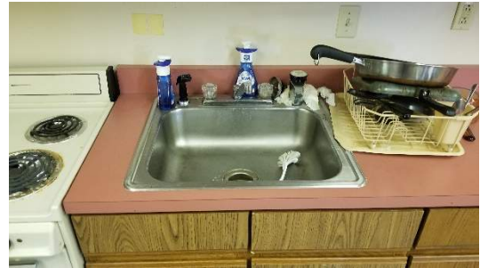
Kitchen Sink with Sprayer and Hot Water Dispenser
