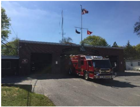
Building Exterior facing High Street
