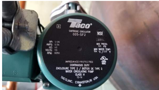
Circulating Pump Nameplate
