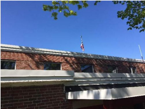
Roof edge and metal coping
